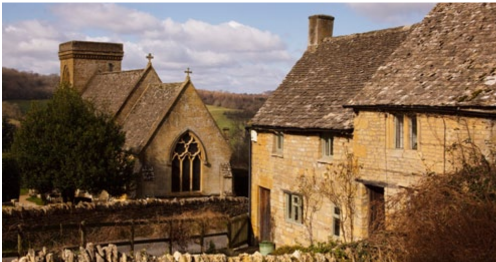
An example of the locally distinctive quarried stone used for domestic architecture at Snowhill, Gloucestershire.
