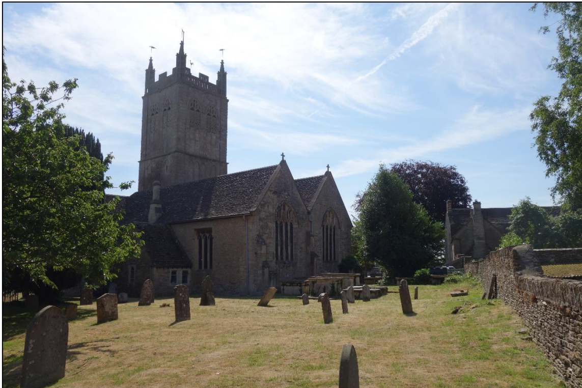
Plate 8: View looking SE across W half of churchyard showing tower and W end of Holy Cross church
