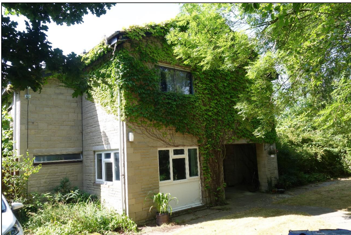
Plate 1: View S towards frontage of existing Vicarage house S of Green Lane, built in 1969
